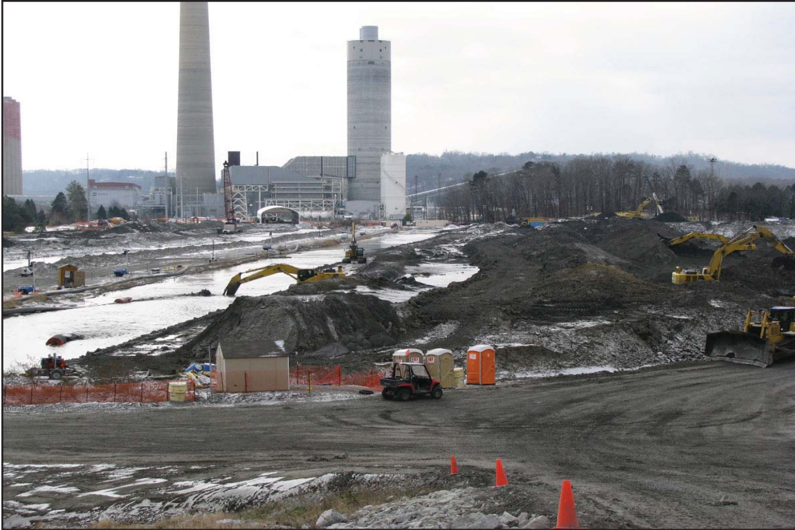
3E - Dipping from Rim Ditch (left) to Ball Field windrows (right). January 8, 2010.
