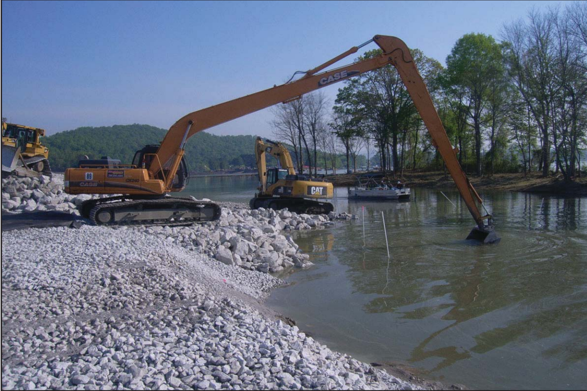
8G - Below water excavation and sand, gravel, and riprap placement. April 23, 2010.
