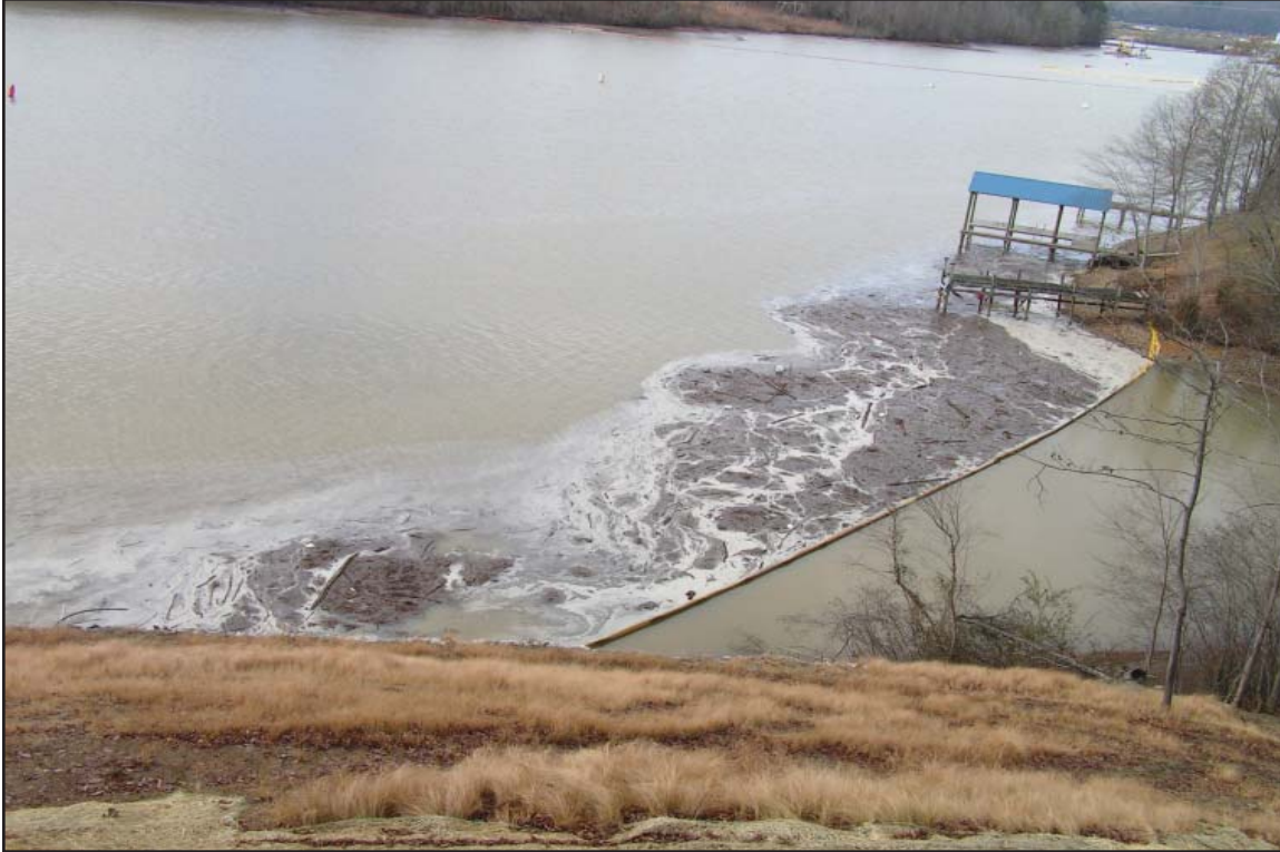
7A - Floating boom used to trap cenospheres and entrained debris on the Emory, Clinch, and Tennessee Rivers. January 23, 2010.
