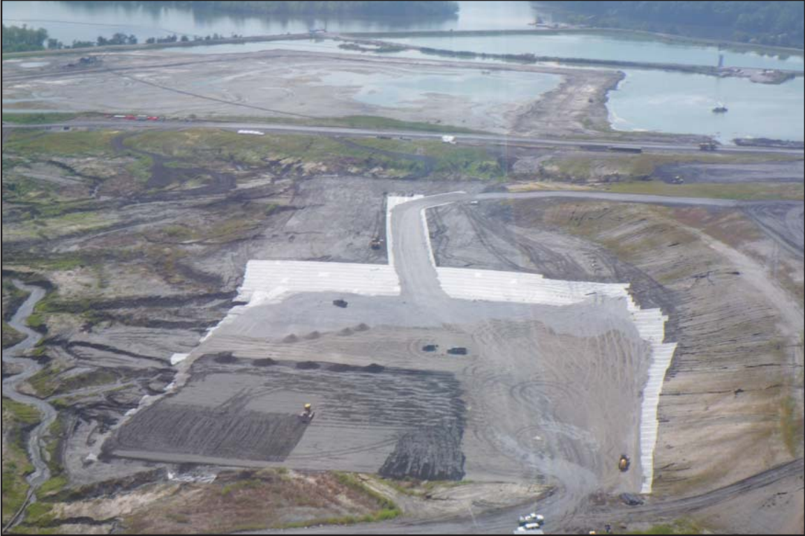
5C - Test embankment, temporary storage of dry-stacked material in test fill. August 10, 2009.
