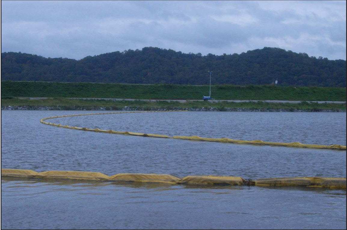
2U - Debris boom downstream of dredging used to collect cenospheres or debris. October 17, 2019.
