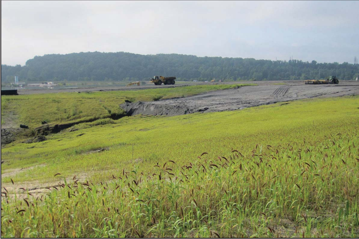
10G - Grass stand following application of Flexterra® by hydroseeding. August 1, 2009.
