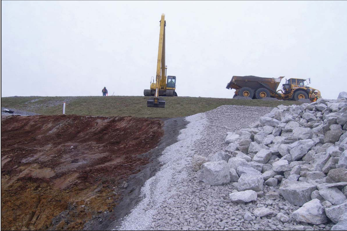
8E - Excavation of subsequent panel next to a completed panel. February 12, 2010.
