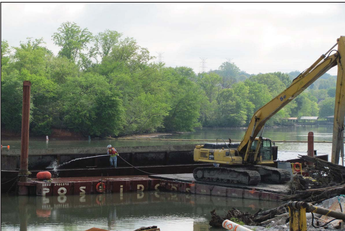
2T - Shore offloading of mechanical dredge barge. April 21, 2010.
