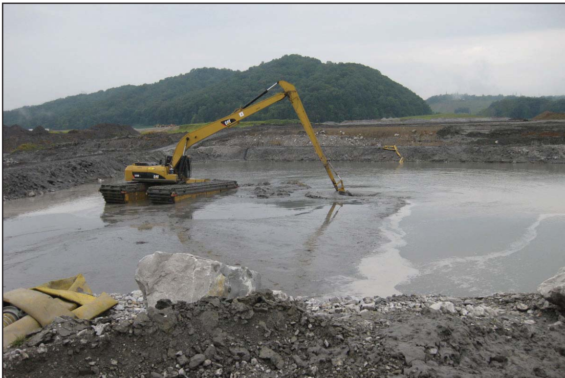
10D - Cleaning out accumulated sediment from the sediment basins. September 4, 2009.
