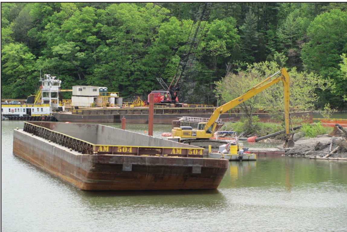
2R - Aquarius mechanical dredging. April 15, 2010.
