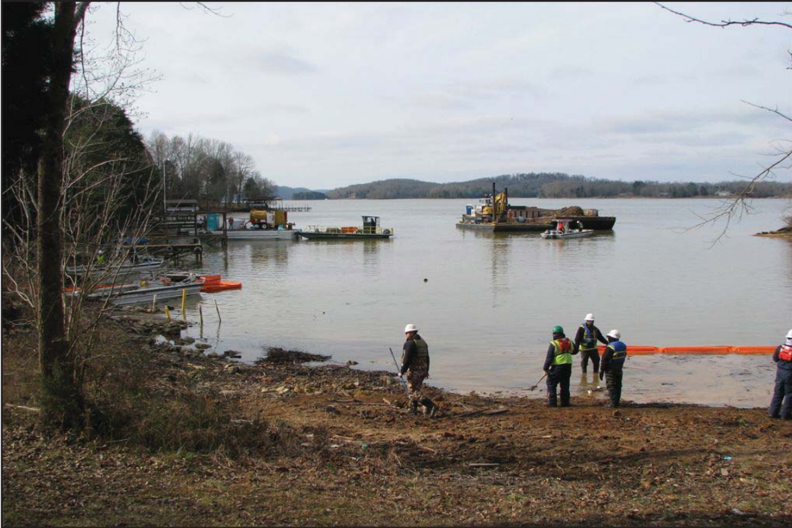
7G - Shoreline debris removal on the Tennessee River. February 12, 2010.
