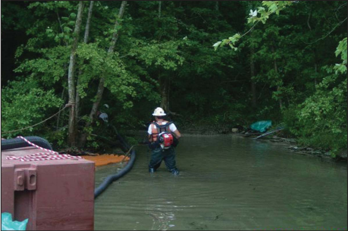
7E - Vacuum removal of cenospheres into holding tank. July 14, 2009.
