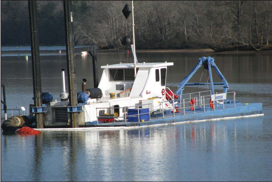
2C - Sevenson Kylie 16-inch dredge (Phase 1 dredging). December 17, 2009.
