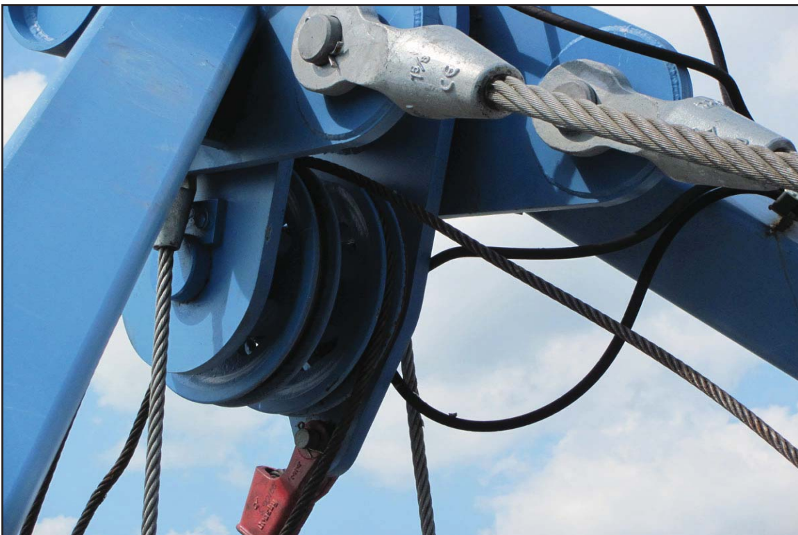
2N - Dredge boom, hydraulic lines, and cables. May 22, 2010.
