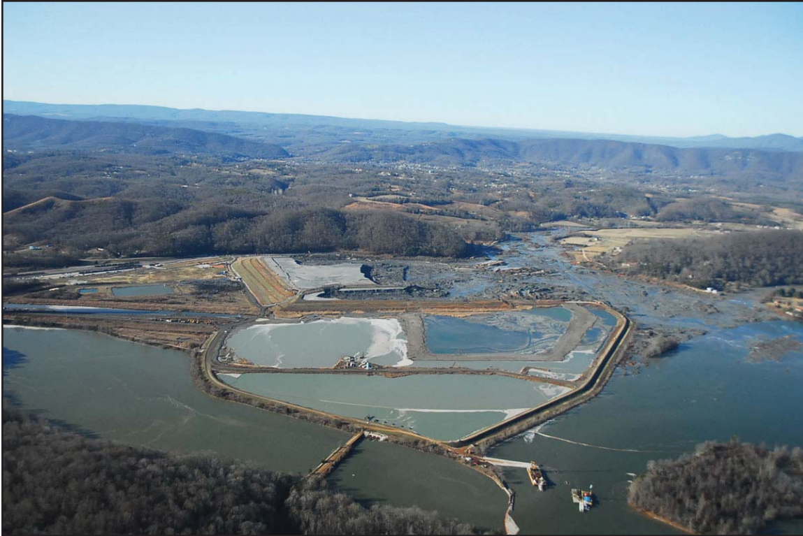
1A - Oblique of the Kingston Ash Recovery Project site after release (viewing from the east). December 29, 2008.
