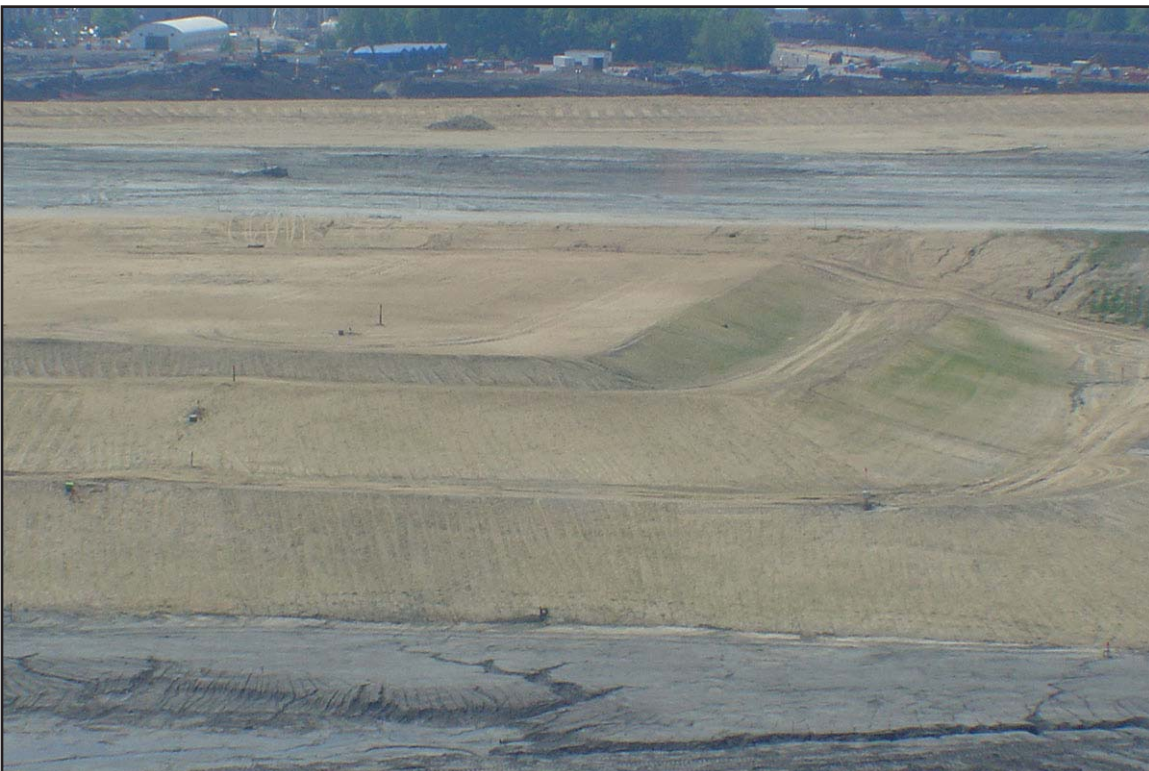
9H - Completed test embankment showing final benched slopes. May 2010.
