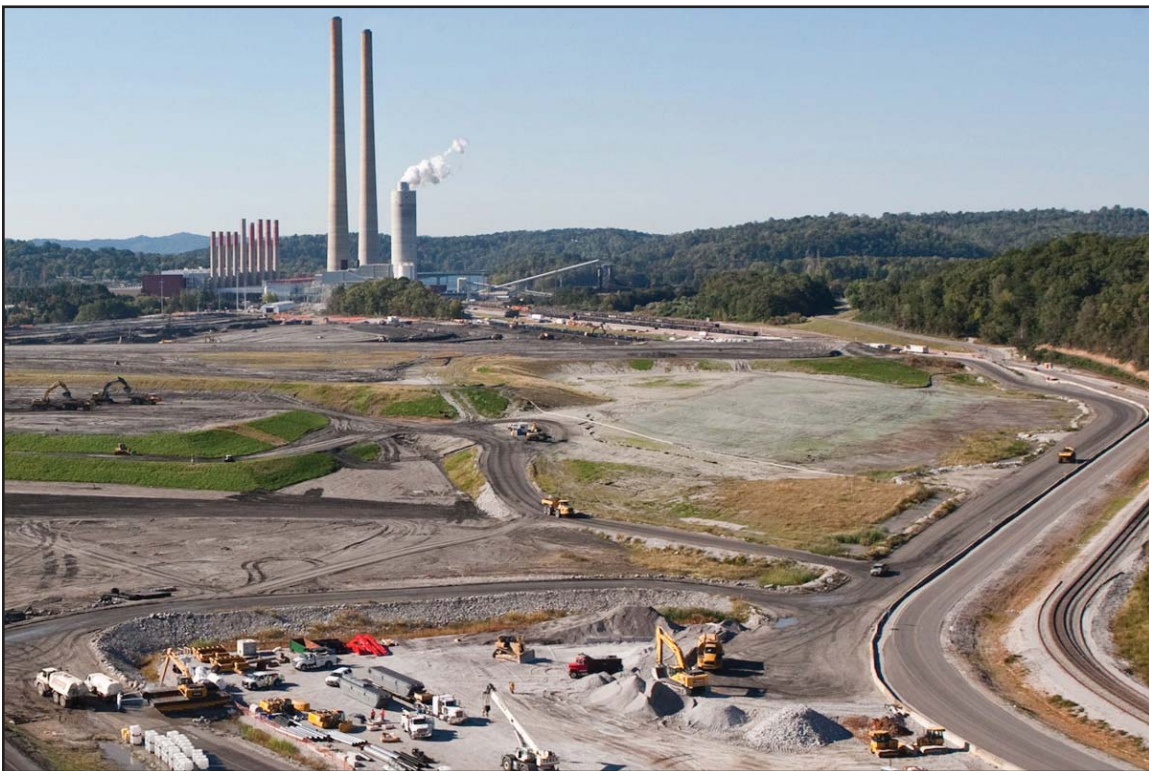
1L - AFTER: Dredge Cell after time-critical removal action. May 7, 2009.
