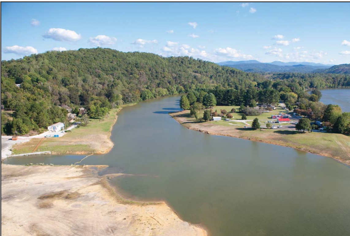
1H - AFTER: East Embayment after time-critical removal action. July 2010.
