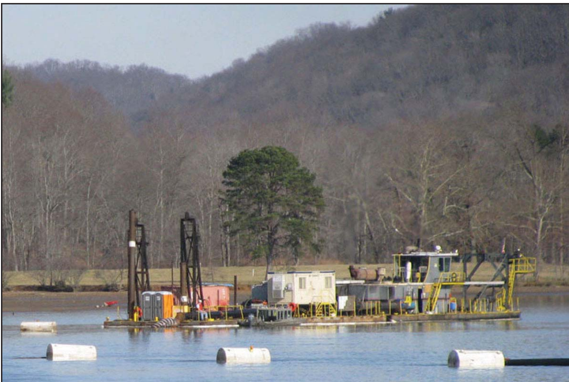
2D - Sevenson Sandpiper 20-inch dredge (Phase 1 dredging). December 17, 2009.
