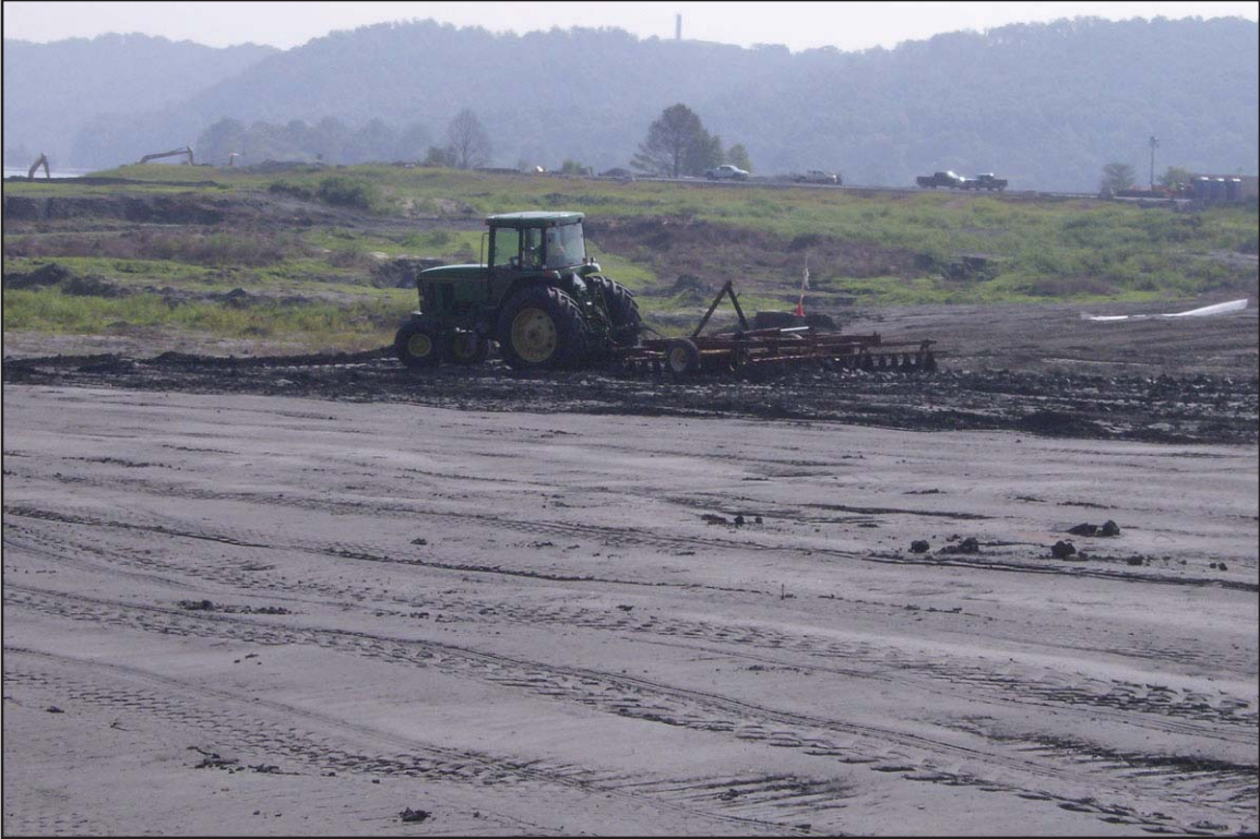
9C - Disking ash in lifts for moisture conditioning. August 14, 2009.
