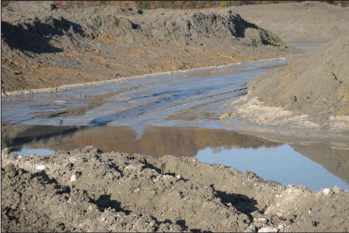
10A - Dirty water ditch used to convey stormwater in contact with exposed ash on the site. November 5, 2009.
