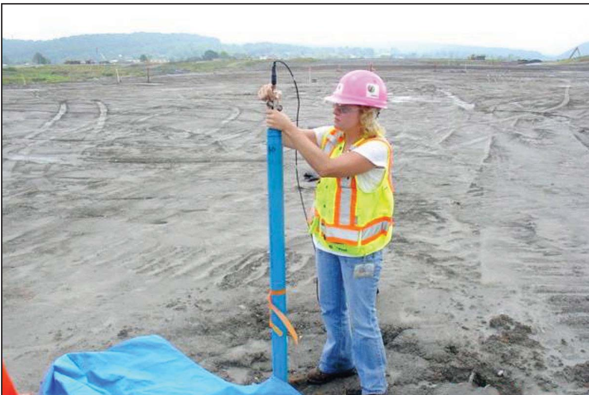
9F - Monitoring of inclinometer instrumentation. August 13, 2009.
