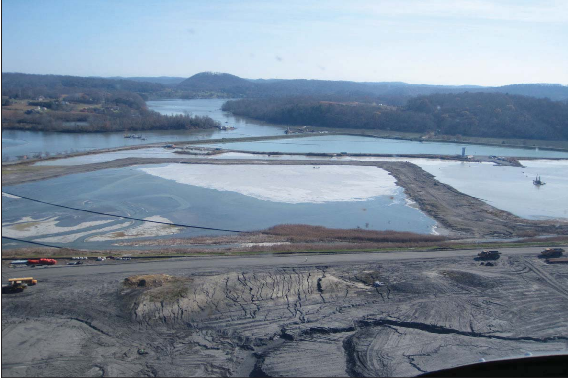
3M - Lateral Expansion Area prior to use for ash recovery. November 20, 2009.
