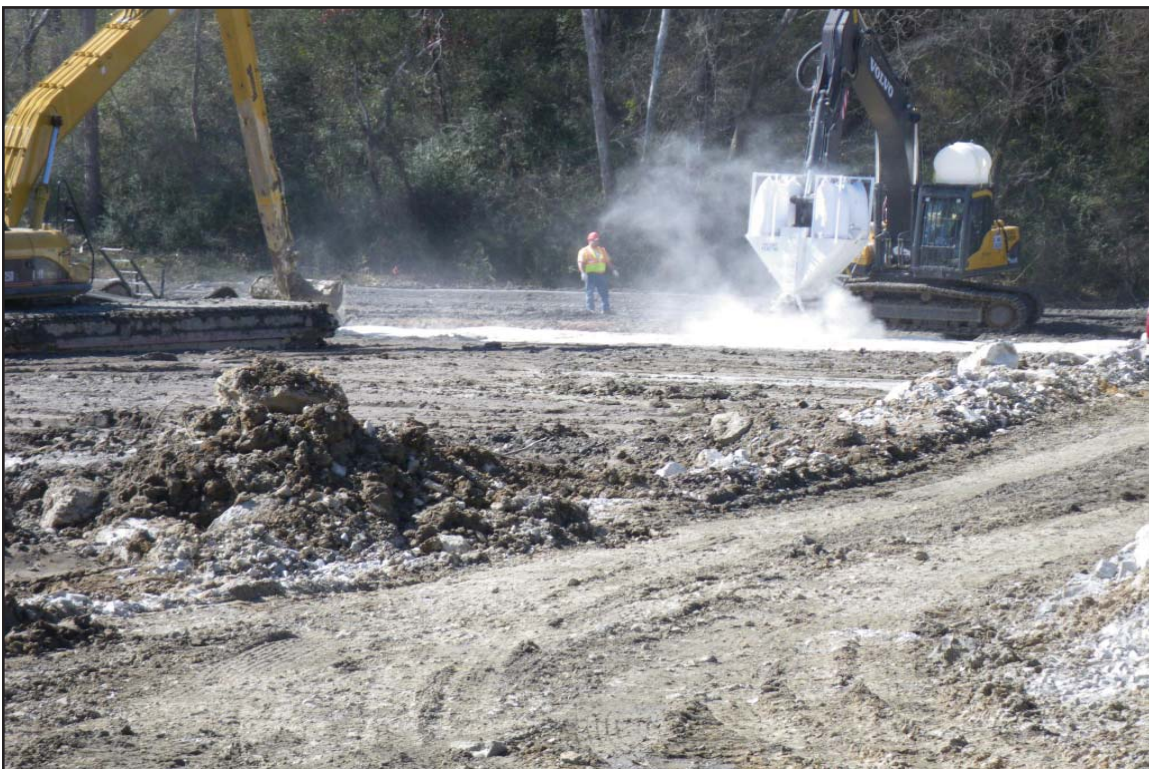
4P - Addition of lime to surface of excavation. March 4, 2010.
