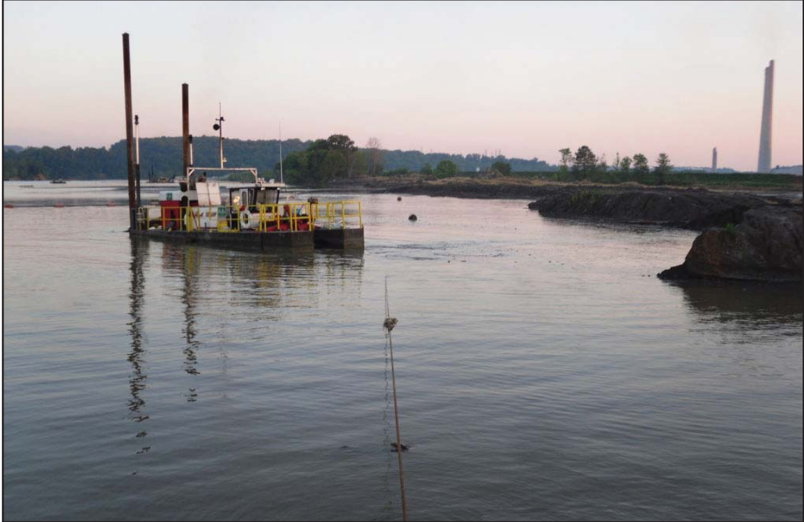
2A - TransAsh Emory dredge operating in the Emory River at the mouth of the clear water ditch. June 24, 2009.
