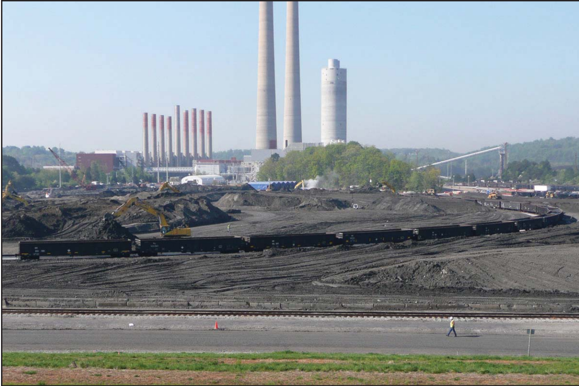
6A - Completed center rail spur in the Ball Field. April 14, 2010.
