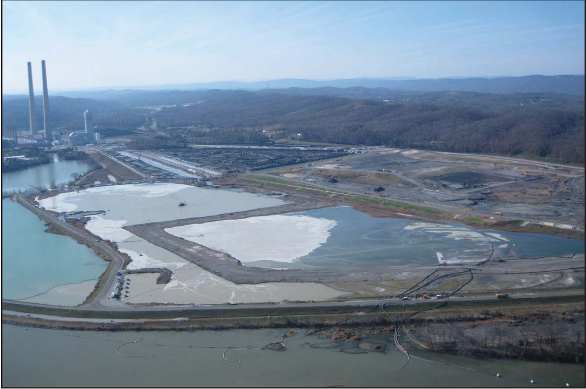
3K - Water treatment in settling ponds, including Ash Pond (top), Stilling Pond (left), and Lateral Expansion (right). November 20, 2009.
