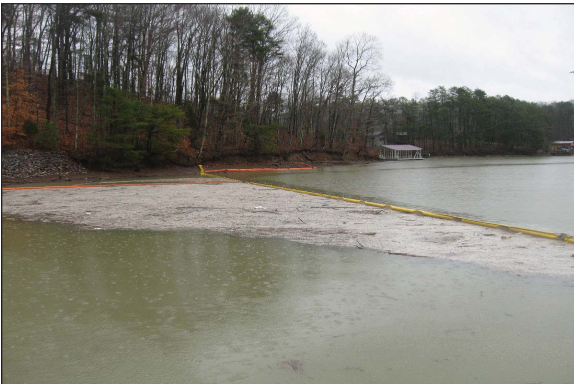
7B - Floating boom used to trap cenospheres and entrained debris on the Emory, Clinch, and Tennessee Rivers. January 24, 2010.
