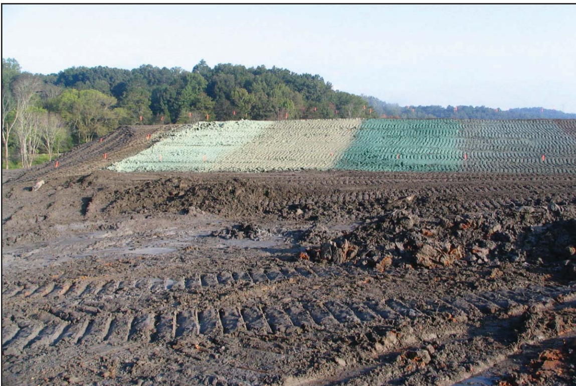
10F - Test plot of hydroseeded formulations to control erosion and reduce dust. September 3, 2009.
