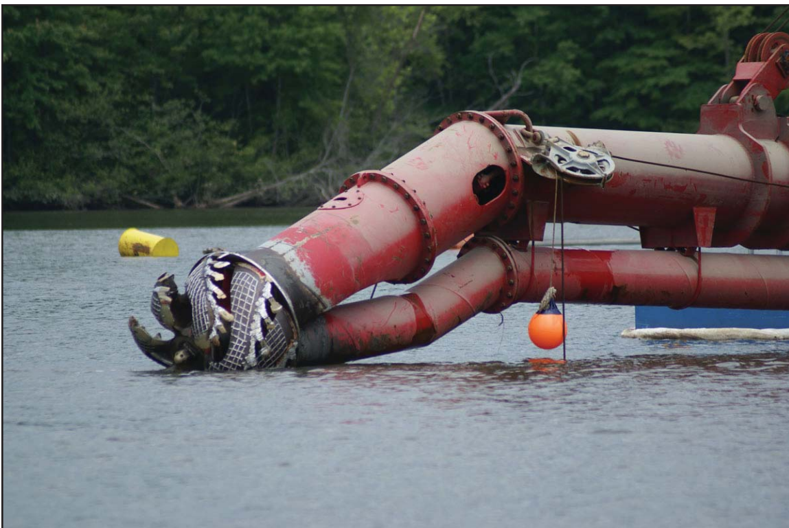
2J - Severson 16-inch cutter head and boom for shallower cut. May 18, 2010.
