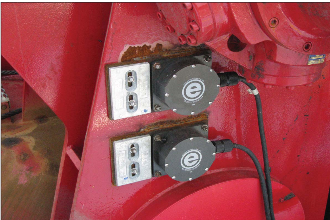
2L - GPS equipment onboard dredge used to guide precision dredging. June 3, 2010.
