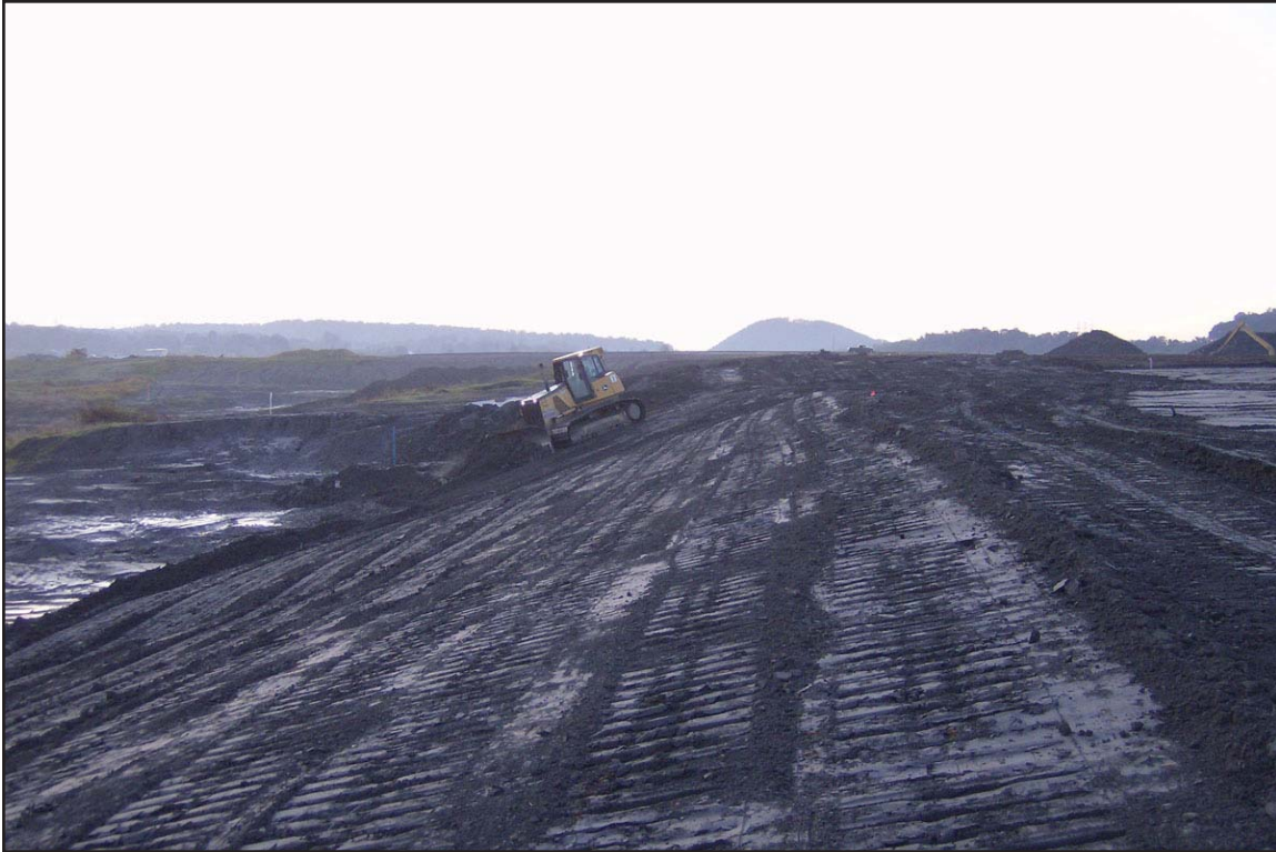
9E - Shaping of side slope of test embankment. September 30, 2009.
