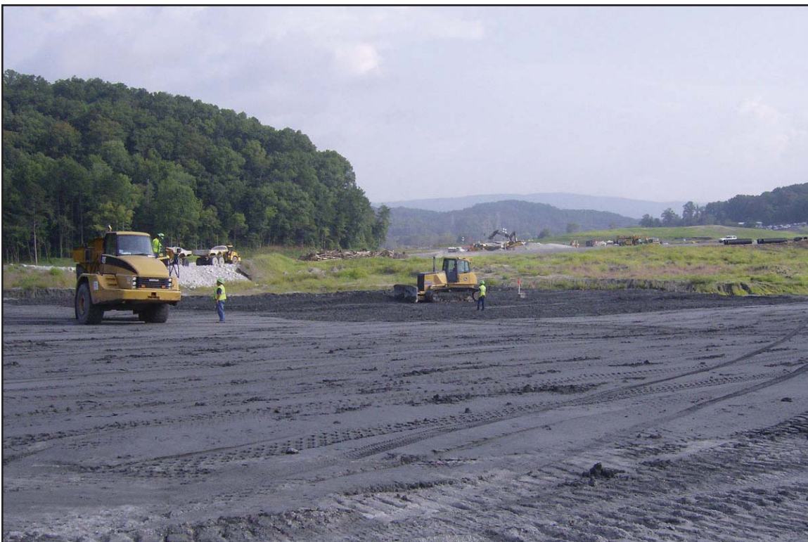
9B - Placing initial lifts within the embankment. August 11, 2009.
