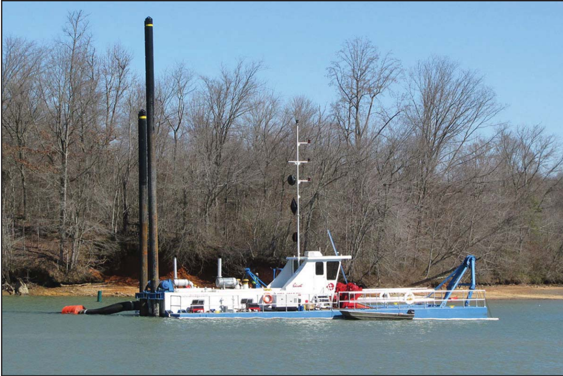
2E - Sevenson Shirley 16-inch dredge (Phase 2 dredging). February 26, 2010.
