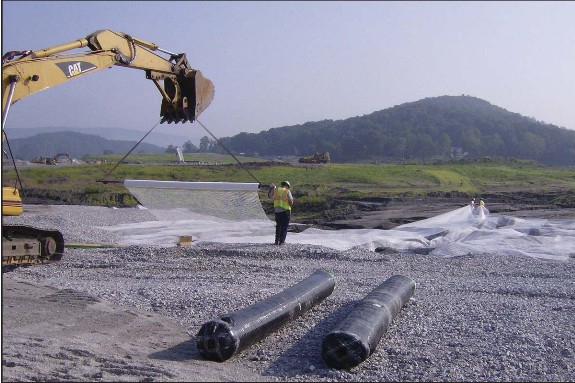
9A - Preparing subgrade (placing geogrid reinforcement and stone). August 7, 2009.
