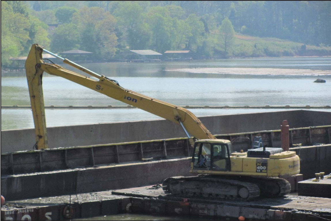
2S - Aquarious mechanical dredging. April 15, 2010.
