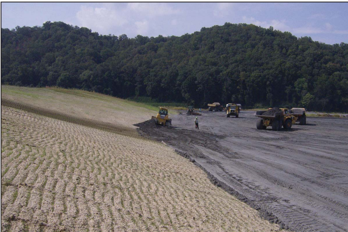
9D - Filling embankment against former relic dike. September 14, 2009.
