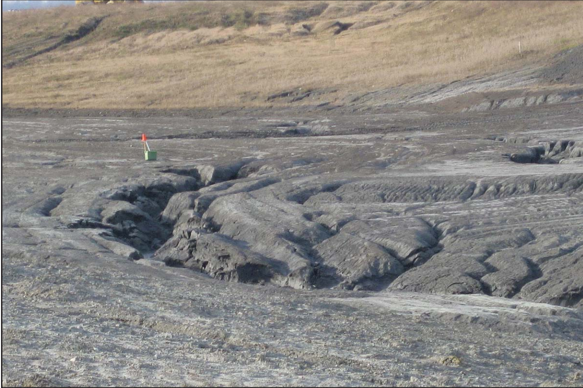
10E - Erosion gulleys that formed in exposed ash following a storm event. December 16, 2009.
