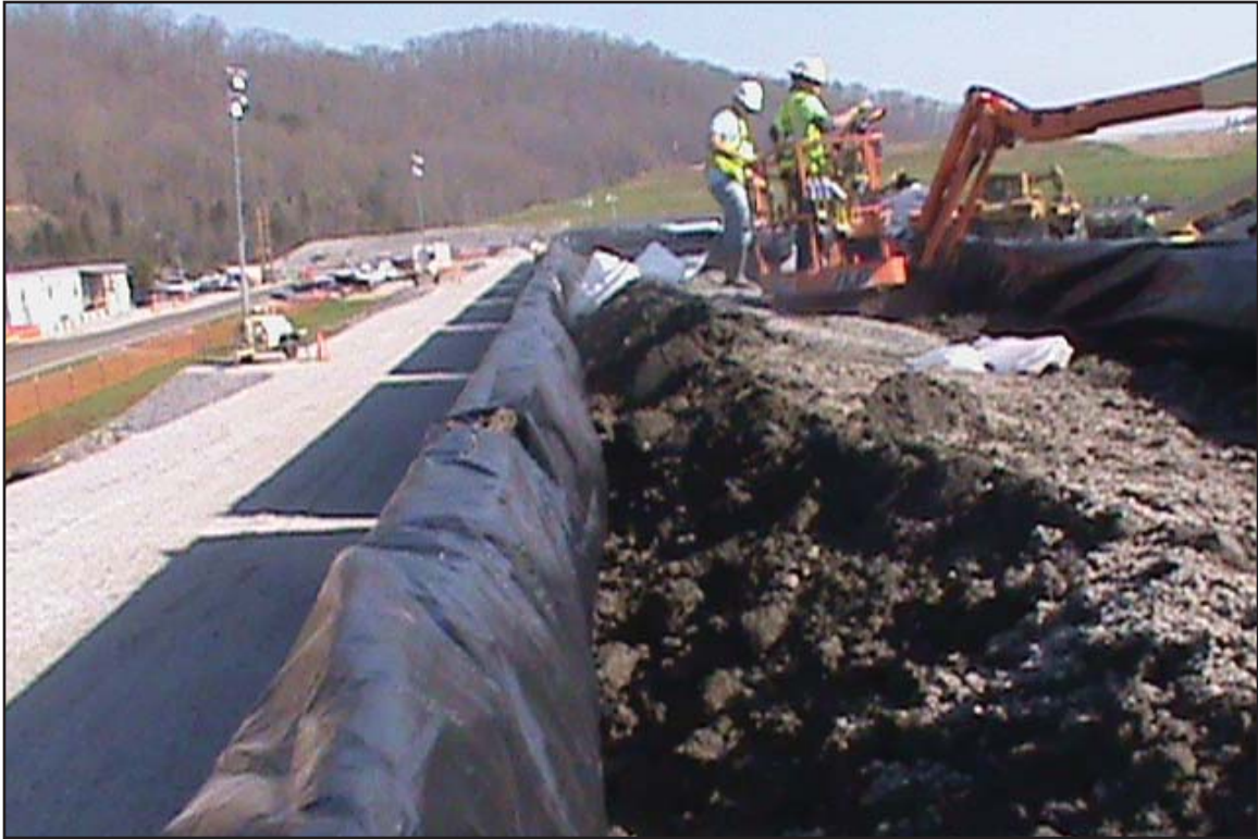
6C - Cherry picker inspecting "burrito bags" in railcars. April 1, 2010.
