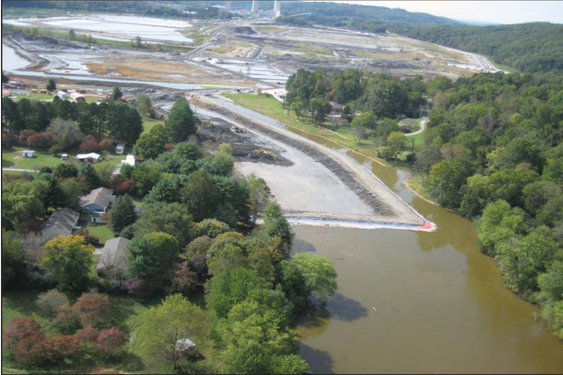
4M - Excavation in East Embayment area with portadam containment. October 8, 2009.
