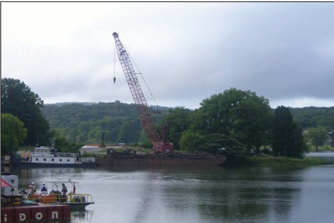
7H - Shoreline debris removal using crane. July 13, 2009.
