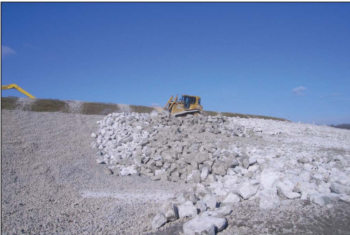
8D - Placing riprap on top of gravel material. December 27, 2009.
