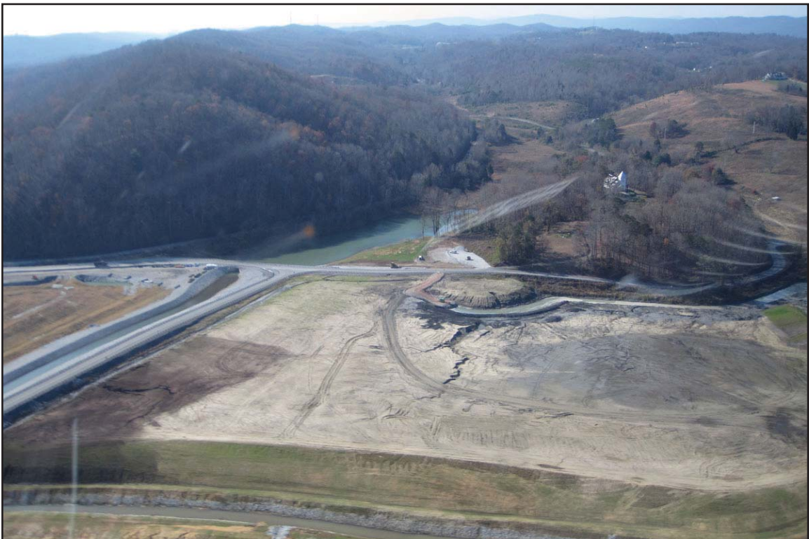
1J - AFTER: North Embayment after time-critical removal action. November 20, 2009.
