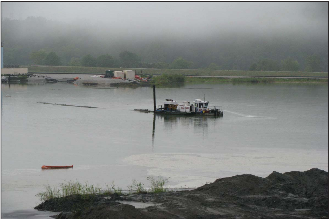
3L - Dredging of Ash Pond to remove settled ash and increase available free water volume. August 15, 2009.
