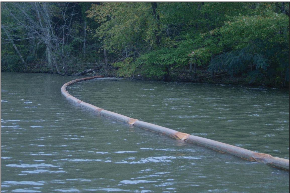
2V - Debris boom downstream of dredging used to collect cenospheres or debris. October 17, 2019.
